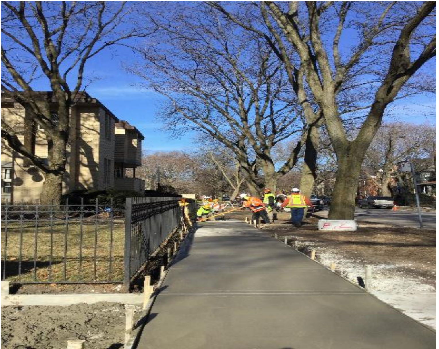
South District - Concrete Sidewalk Restoration
